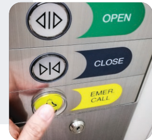
Elevator Call Box
